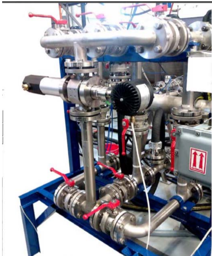
Figure 1. Canty InFlow, Rig Installation
